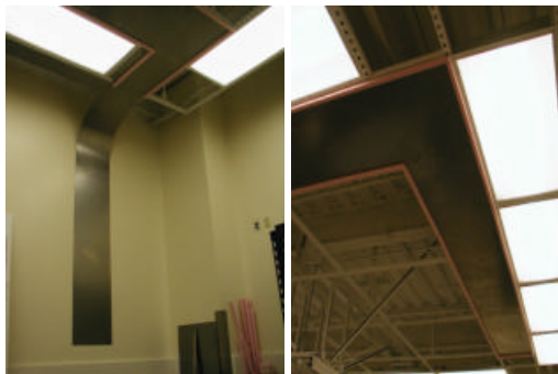
Fig. 7: Demonstration Magnebot space in CIMIT simulation room: (a) L-shaped ceiling section; (b) Curved transition to vertical wall section.
